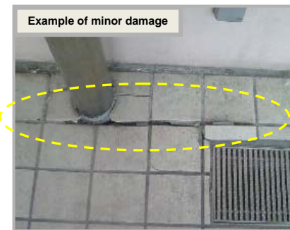
Crack in the tiles around the building
