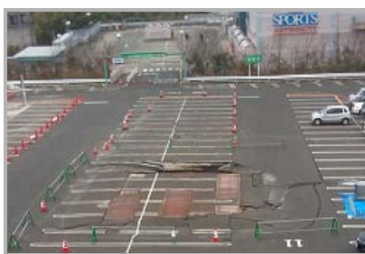
Caving of drain facilities [Parking lot in front of Main building]
