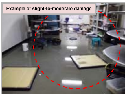
Damage to the equipments in the projection booth due to the activation of the fire sprinkler
