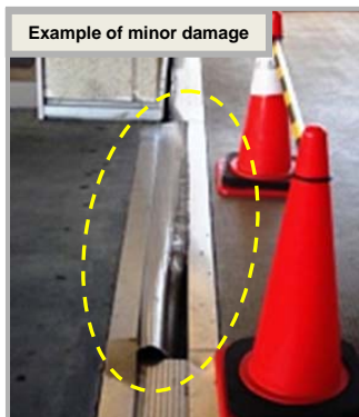
Damage to the cover of the joint section between buildings
