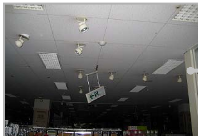
Damages to ceiling facilities [2F Main building]
