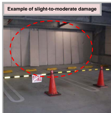
Inward dislocation of the exterior wall of the parking building
