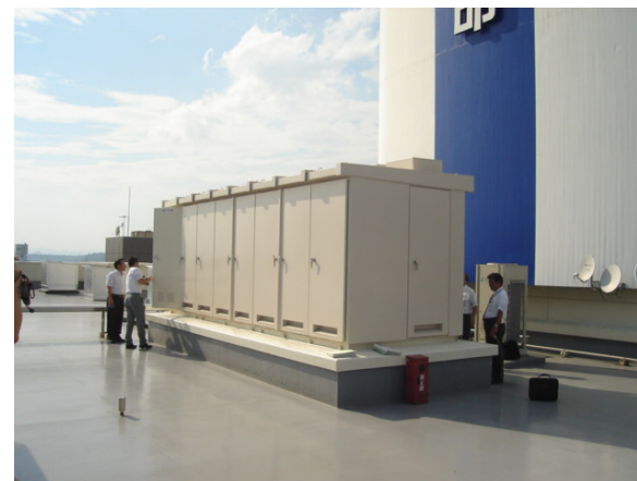
Southern Mito Building
