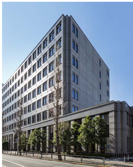
Sasazuka Center Bldg.
