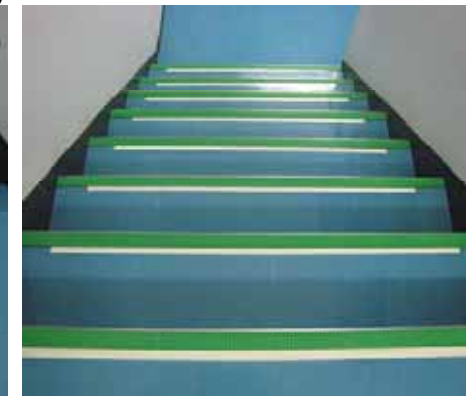
Installed handrails and luminous tape on emergency staircases
