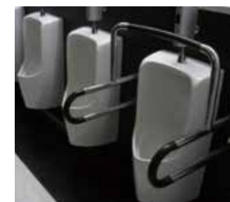
Installation of handrails
