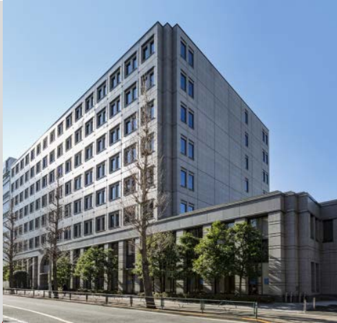
Sasazuka Center Bldg.
