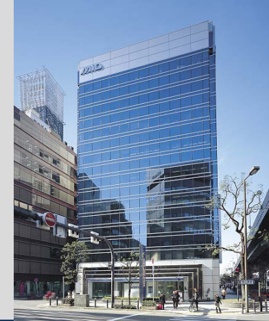
MID Nishihommachi Bldg.
